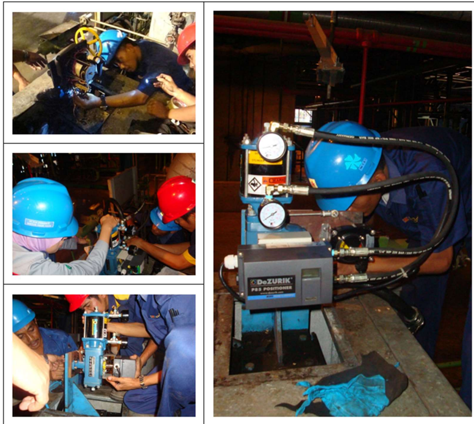
Gambar 9. Proses Retrofit Speed Control Actuator BFP 1A
