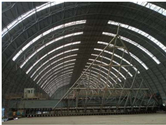
Gambar 2. Bridge type reclaimer limestone
