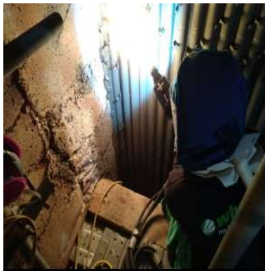
Gambar 7. Proses metal coating
