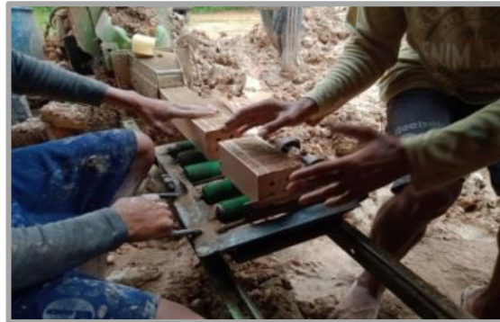
Figure 6. Brick Cutting
