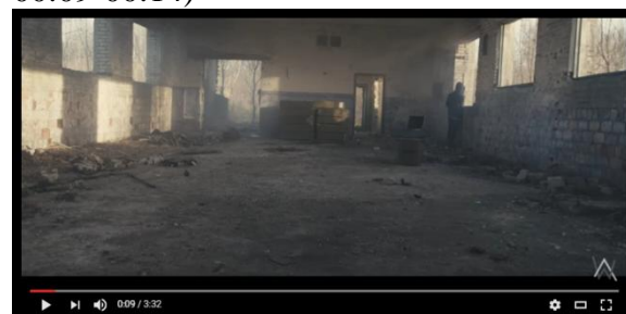
Figure 4. The devastated house
